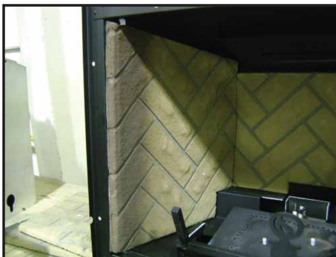
Figure 3. Install Side Refractory
